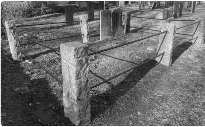
Restoration of Central Cemetery — all new wrought iron and new granite post
